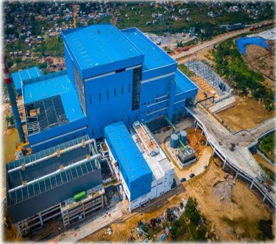
19.8 MW capacity- GHMC
